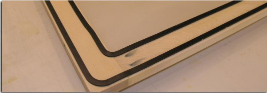
24. Return the frame to its normal use position (with the top face of the frame upward). Apply a bead of silicone caulk to the outer edge of the 4 cleats and smooth it down with [your finger](#) or a smoothing tool. The bead of silicone is the secondary defense against leaks.
